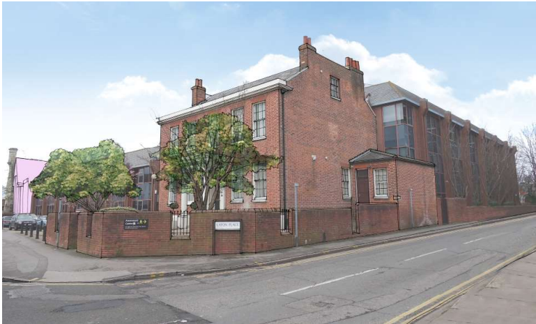
Existing view looking towards Mannson House from Corner of Oxford Road and Eaton Place
