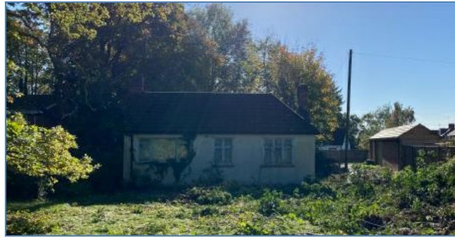
Fig 3. Existing site photo submitted within Stage 2 Report.
