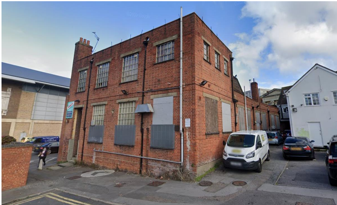
Figure 3 – Street view of the rear elevation of the existing building from Crossland Road (Source: Google Maps)
