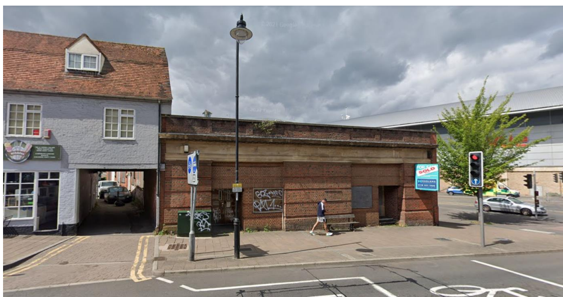
Figure 1 – Street view of the eastern elevation of the existing building, from London Street (Source: Google Maps)
