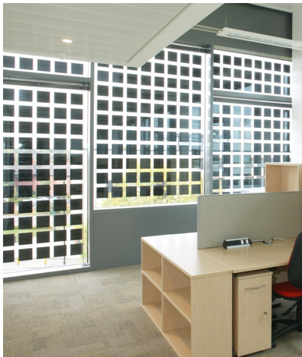
Figure 6 - CPW Solar Glazing Installation, University of Warwick - Materials and Analytical Sciences Building
