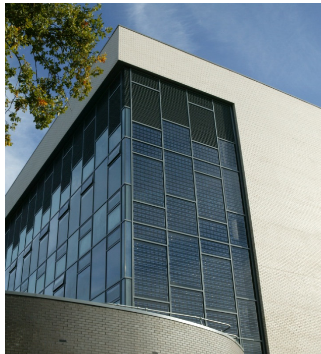
Figure 6 - CPW Solar Glazing Installation, University of Warwick - Materials and Analytical Sciences Building
