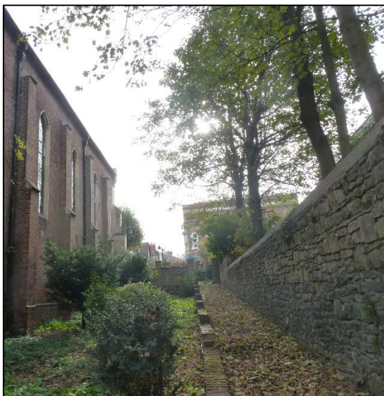
FIGURE 15 LARGE SELF-SEEDED SYCAMORES ARE NOW DAMAGING THE WALLING GA
