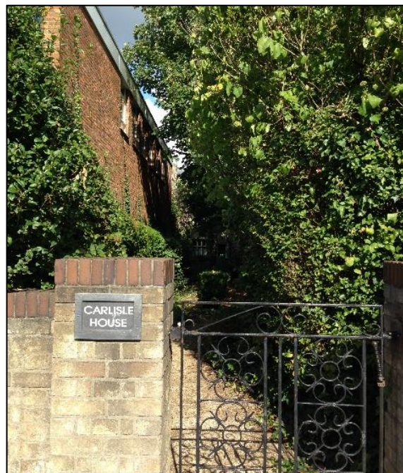
FIGURE 14 EXISTING ENTRANCE TO THE GARDEN FROM OXFORD ROAD IS CURRENTLY MODERN BRICKWORK GA
