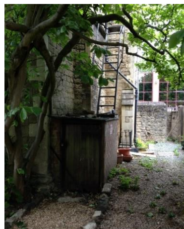
FIGURE 31 MATURE EXISTING MAGNOLIA ON THE SOUTH EAST CORNER OF THE HOUSE TO BE SUPPORTED BY A NEW IRON ARCH GA
