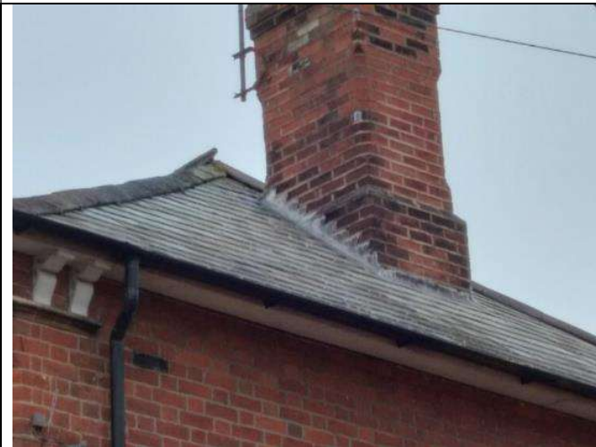
Photograph 2: Close-up of roof on southeast elevation of B1.
