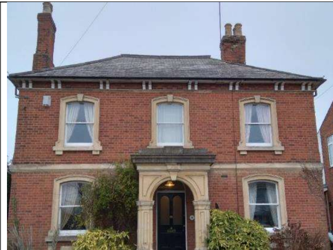
Photograph 1: Southwest elevation of B1.
