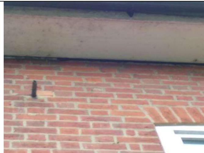
Photograph 4: Close up of soffit box on northeast elevation.
