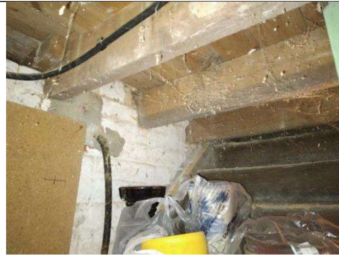
Photograph 15: Space under the stairs which lead into the house.
