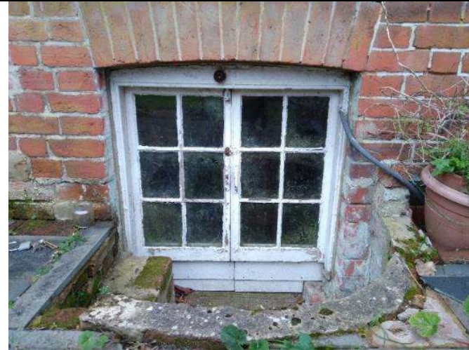
Photograph 8: Basement doors (pictured opposite).
