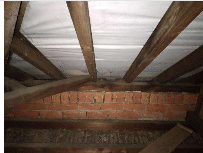
Photograph 9: Interior of eaves space within B1.
