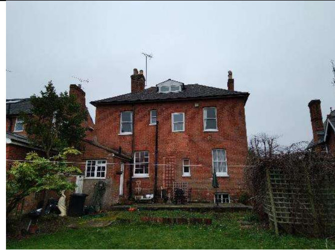
Photograph 16: View of B1 and B2 from the garden.
