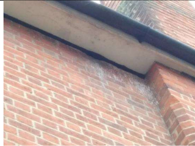
Photograph 7: Close up of the soffit box on the northwest elevation.
