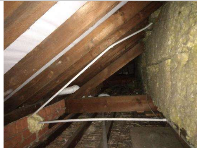
Photograph 11: Eaves space on southwest elevation of B1.
