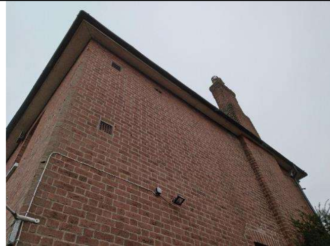
Photograph 6: Northwest elevation of B1.
