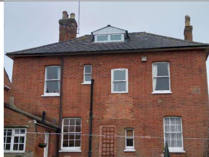
Photograph 3: Northeast elevation of B1.
