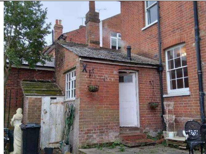
Photograph 5: Single storey extension and brick shed.
