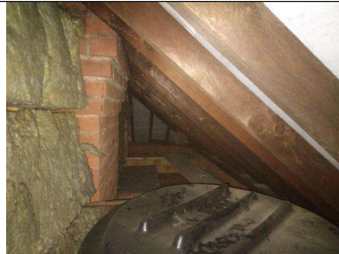
Photograph 10: Eaves space on southeast elevation of B1.
