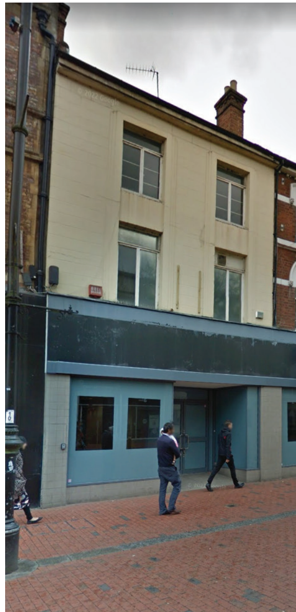
Existing Shop Front
