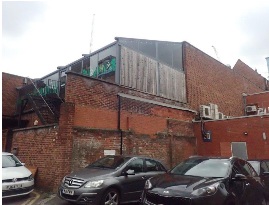
Photograph 5: Rear of buildings at Friar Street, Reading.
