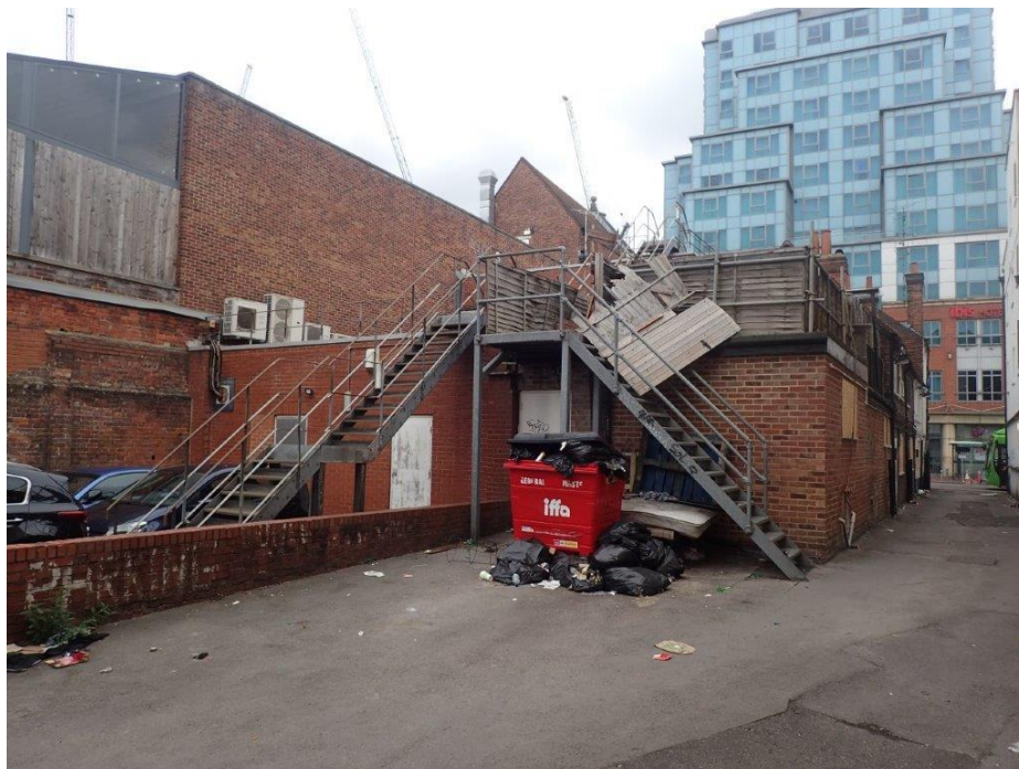
Photograph 6: Rear of the buildings at Friar Street Reading.
