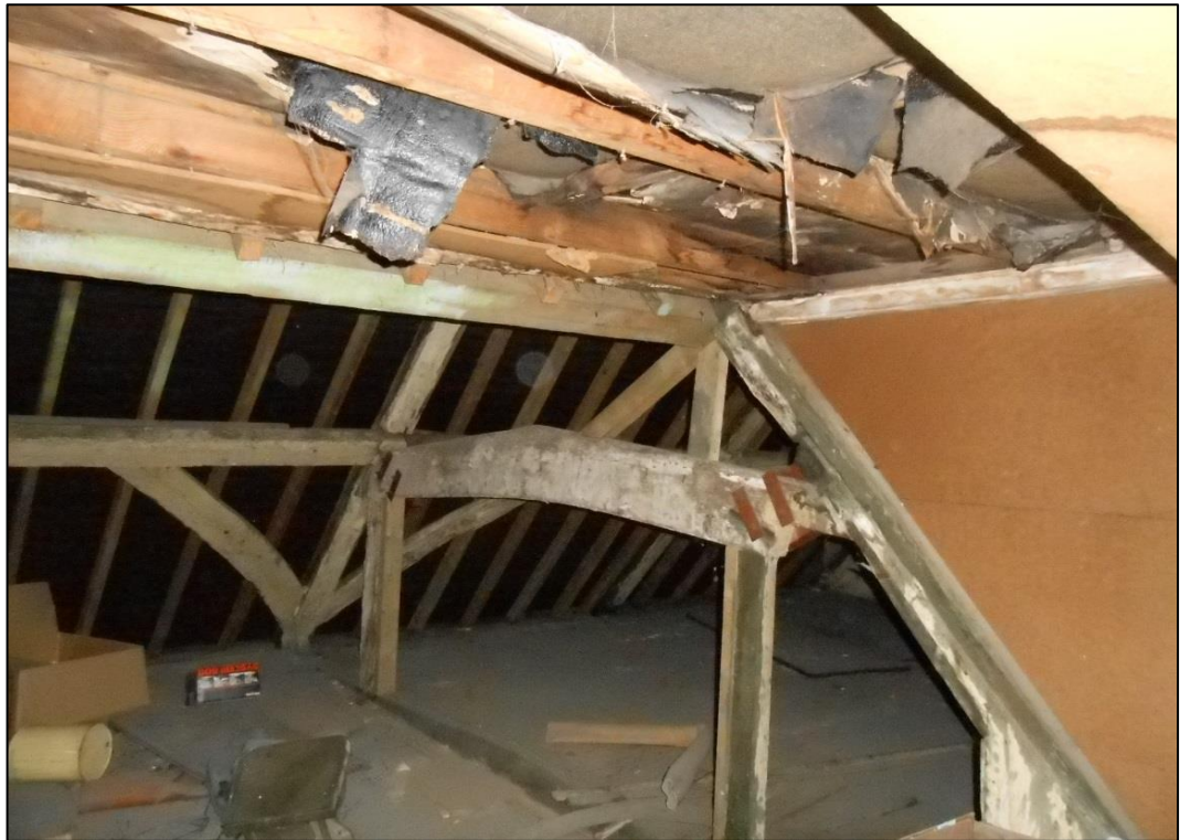
Figure 11: Early to mid-16 th century roof frame. The tie beam can be seen at floor level below the Queen truss.
