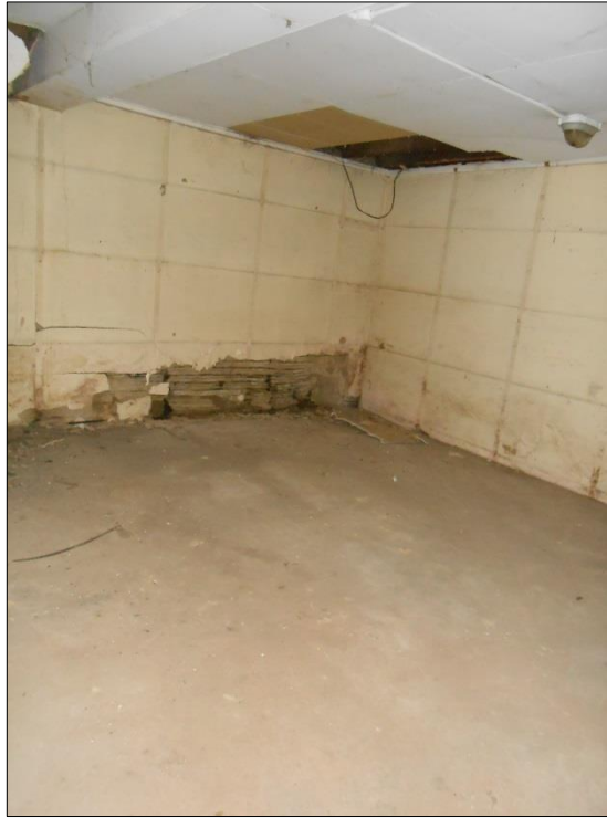
Figure 25: The basement has already been altered.
