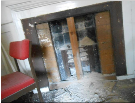
Figure 18: The Victorian fire grate set into the Georgian fire surround
