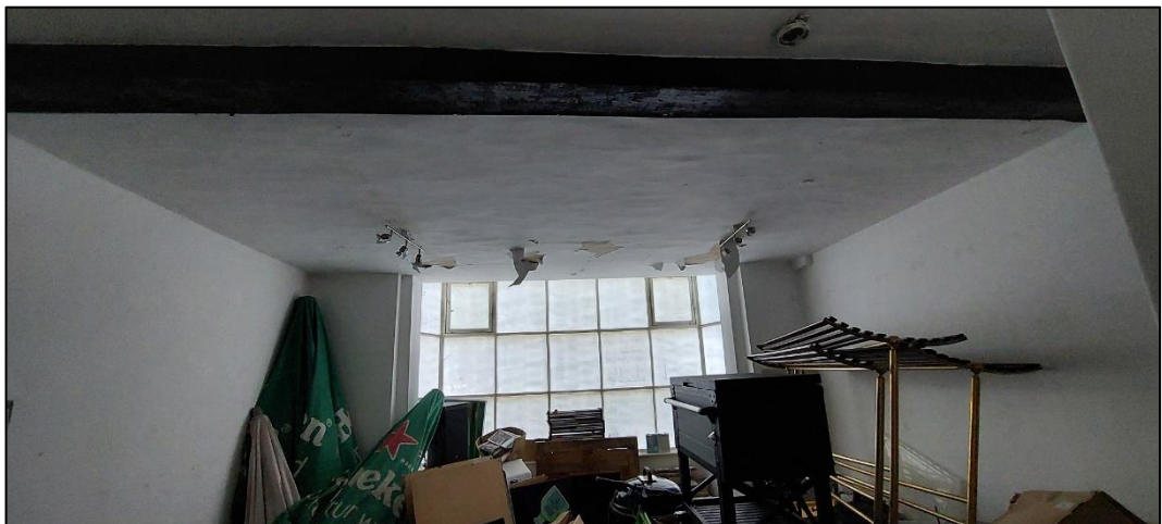
Figure 15: View into right hand 'shop' with single timber being the only feature apart from the window.
