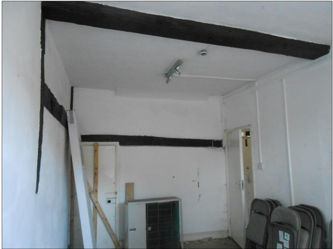
Figure 14: View showing the left hand 'shop' with exposed timber frame. Note the right hand wall is a modern insertion and there is likely to have been a fireplace (now removed) on the back wall (centre)
