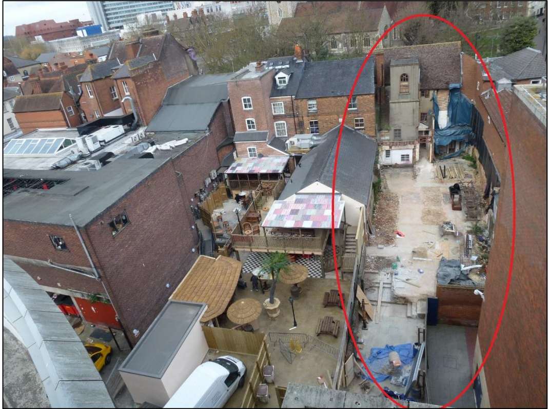
Figure 2: View from elevated vantage point showing the cleared site and back of the historic property
