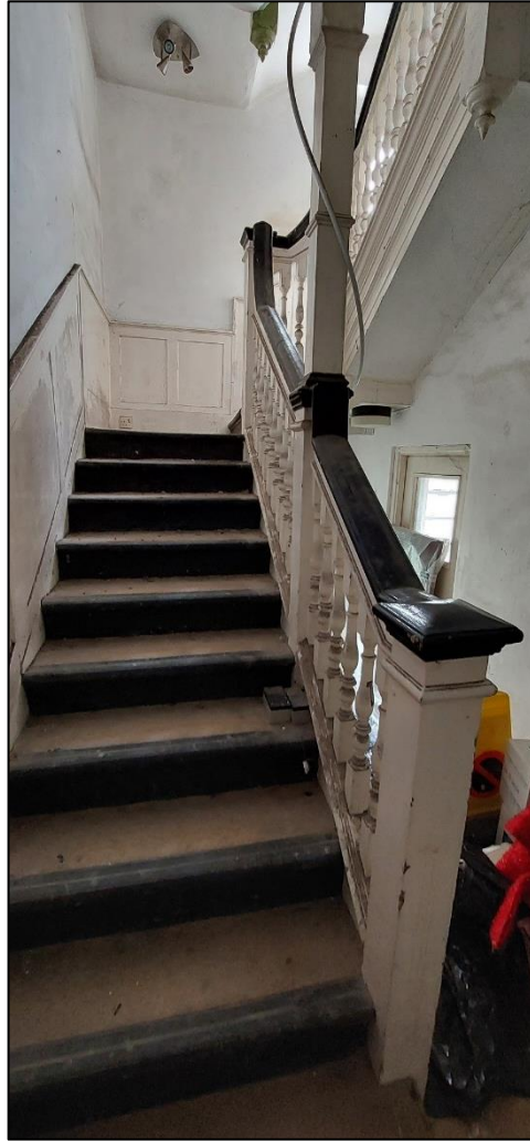
Figure 12: View of staircase
