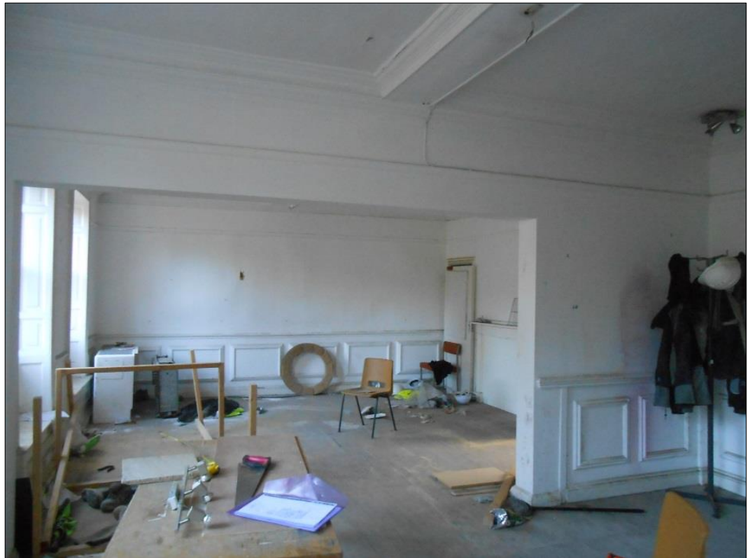
Figure 16: Front first floor rooms have been opened out.
