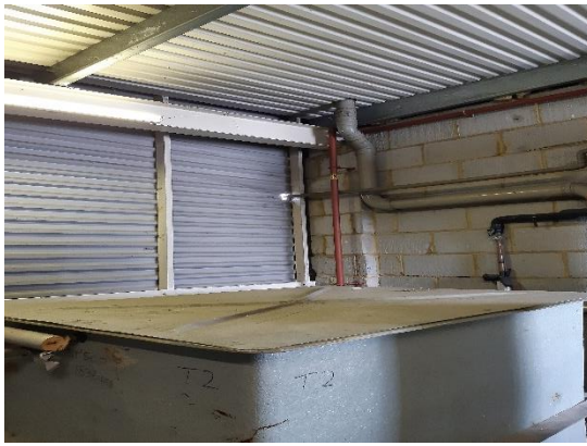
Photo 11: Image taken inside the facilities building on the roof of B1, showing the concrete brick and corrugated metal structure
