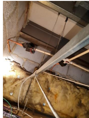
Photo 10: Image taken inside the roof void of B1, between the false ceiling and flat roof, showing insulation present in this area
