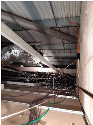
Photo 9: Image taken inside the roof void of B1, between the false ceiling and flat roof
