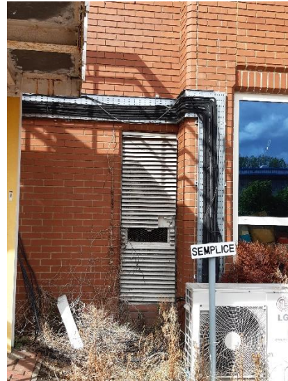
Photo 8: Image taken from the SW of B2, showing the slatted door to the south of the building
