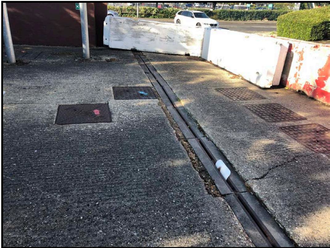
Figure 9 – Existing On-Site Drainage
