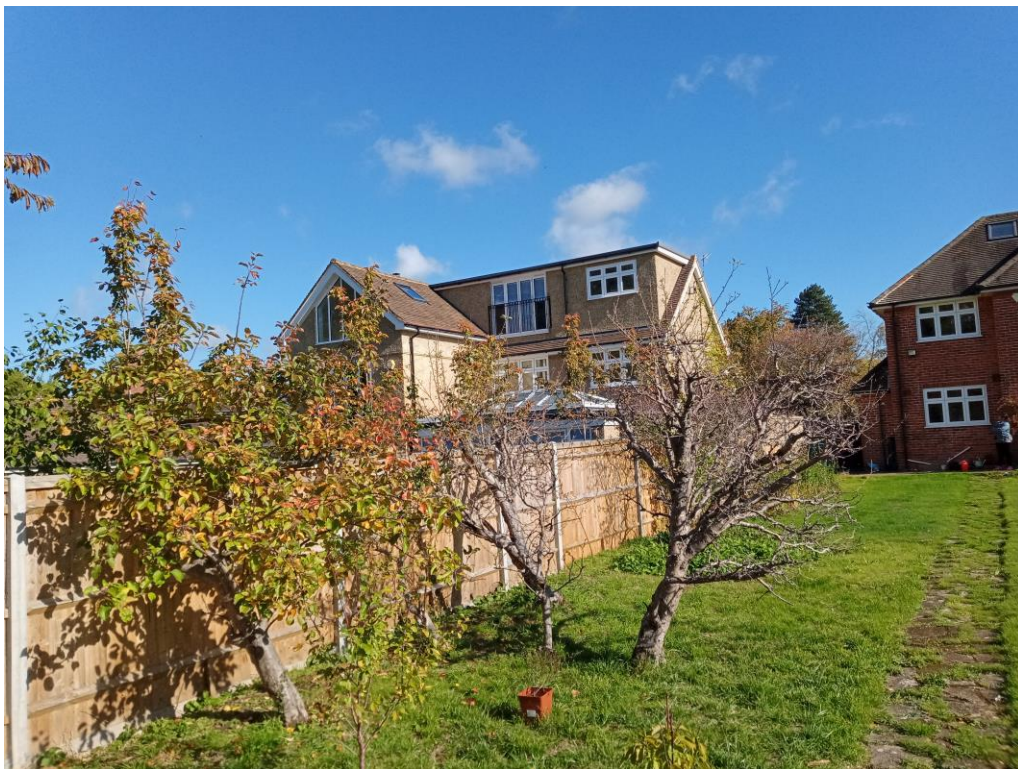
Figure 4: Existing rear elevation no 33 Brooklyn Drive (site visit 10/10/22)
