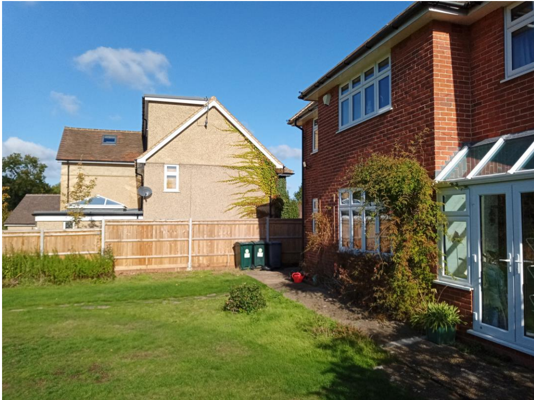
Figure 3: Existing side elevation including flat roof rear dormer at no 33 Brooklyn Drive (site visit 10/10/22)
