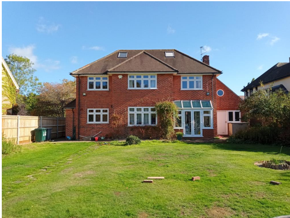
Figure 2: Existing Rear Elevation
