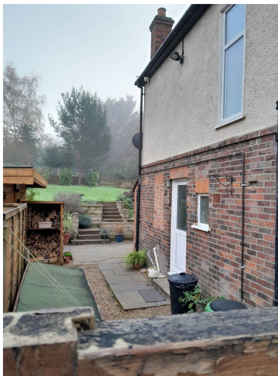
Site visit photo - side elevation
