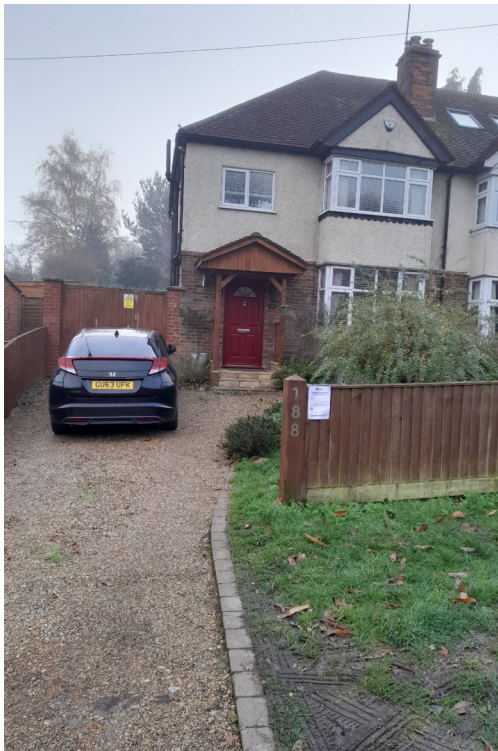
Site visit photo - front elevation
