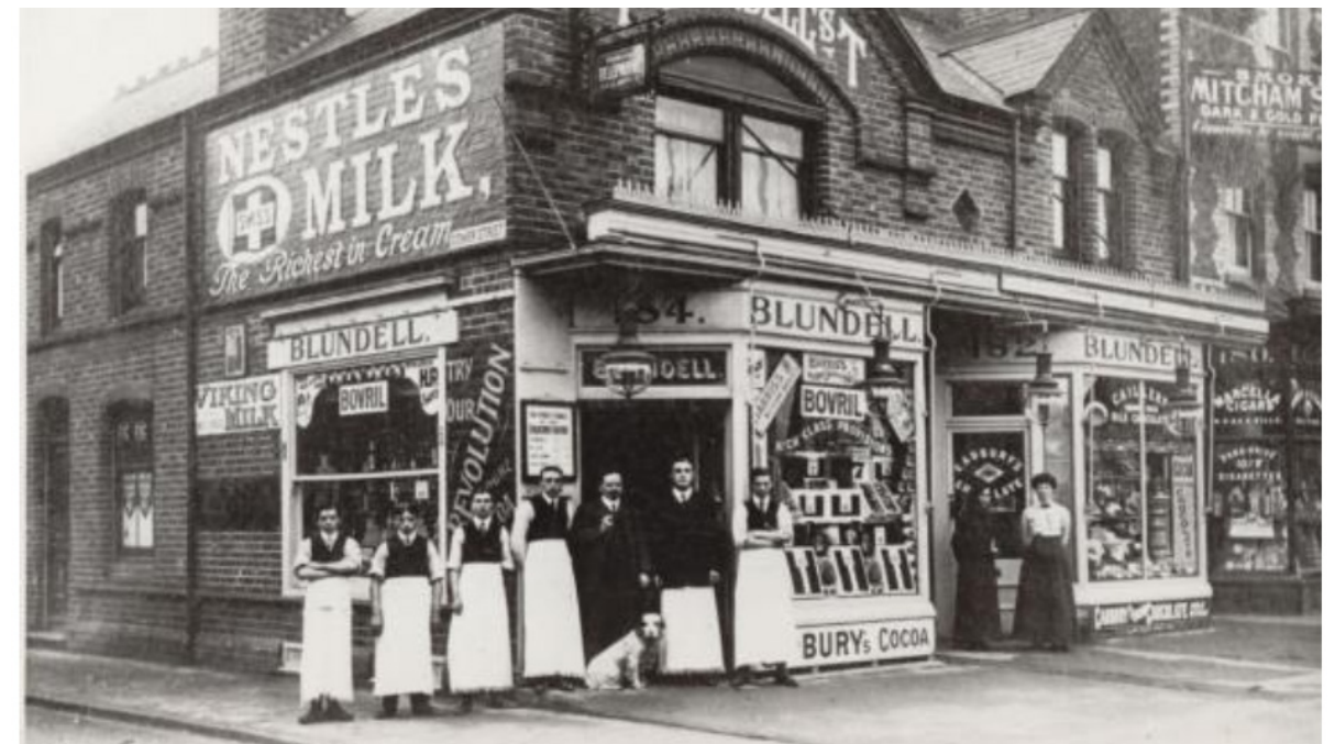
Historical image showing grocery store at no. 184. C. 1910
