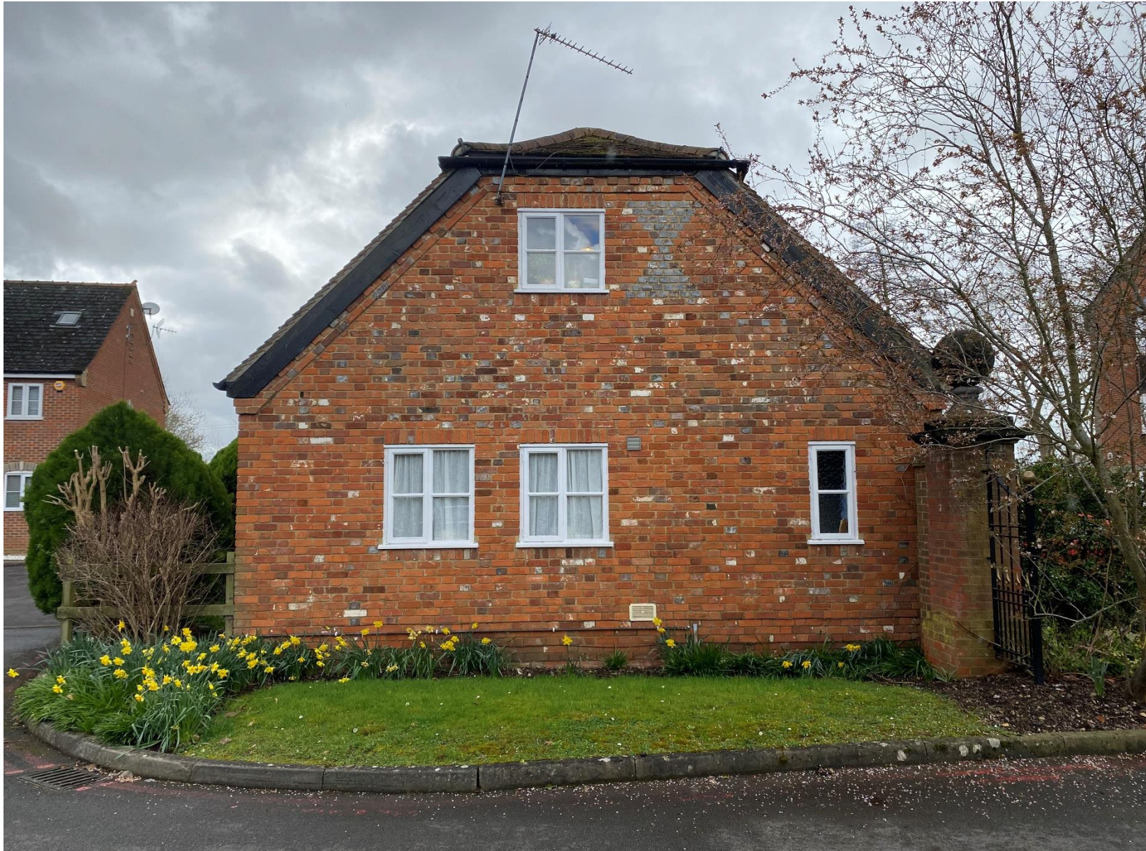
Figure 13 – The Site's north elevation. The proposal location is on this elevation, the pre-existing window and external filters are viewable.
