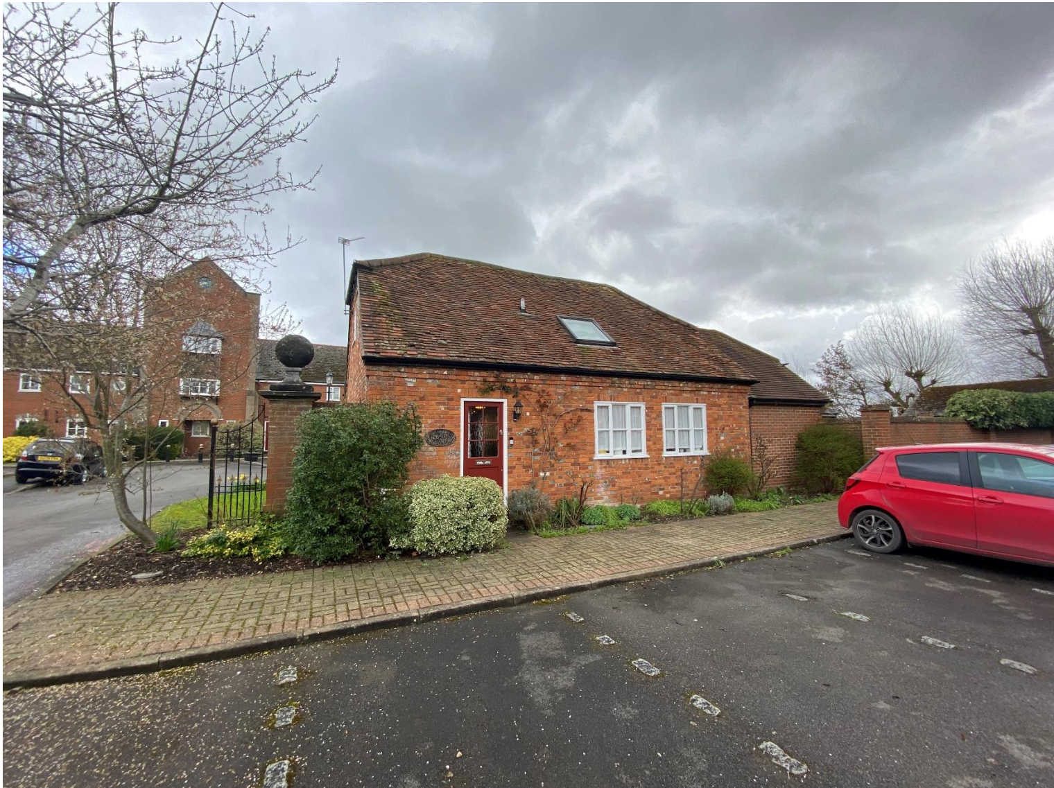
Figure 15 – The Site is in limited scale when compared to neighbouring buildings.
