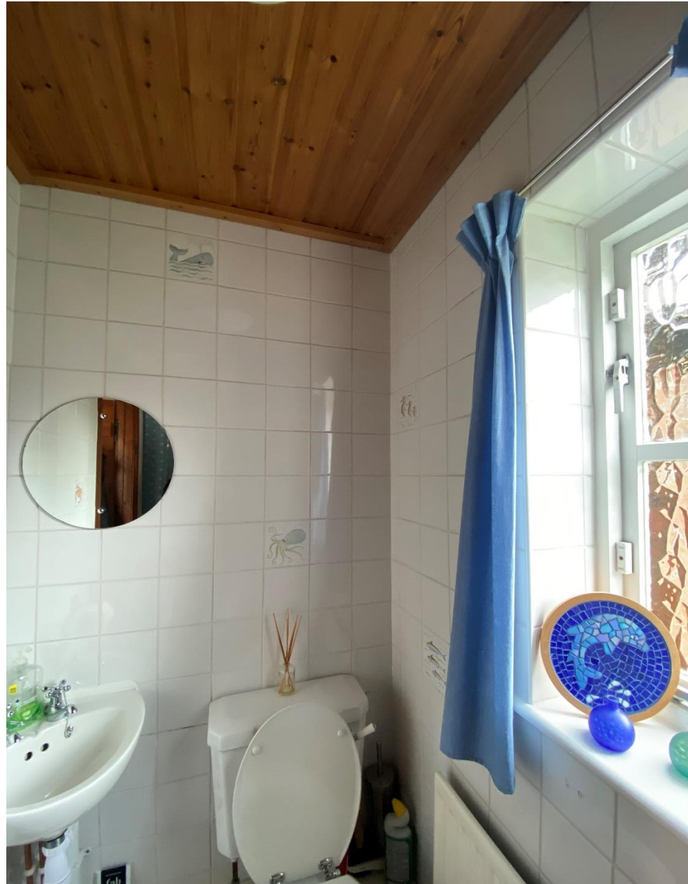
Figure 9 – Alternative view to shower room. Pre-existing window visible.
