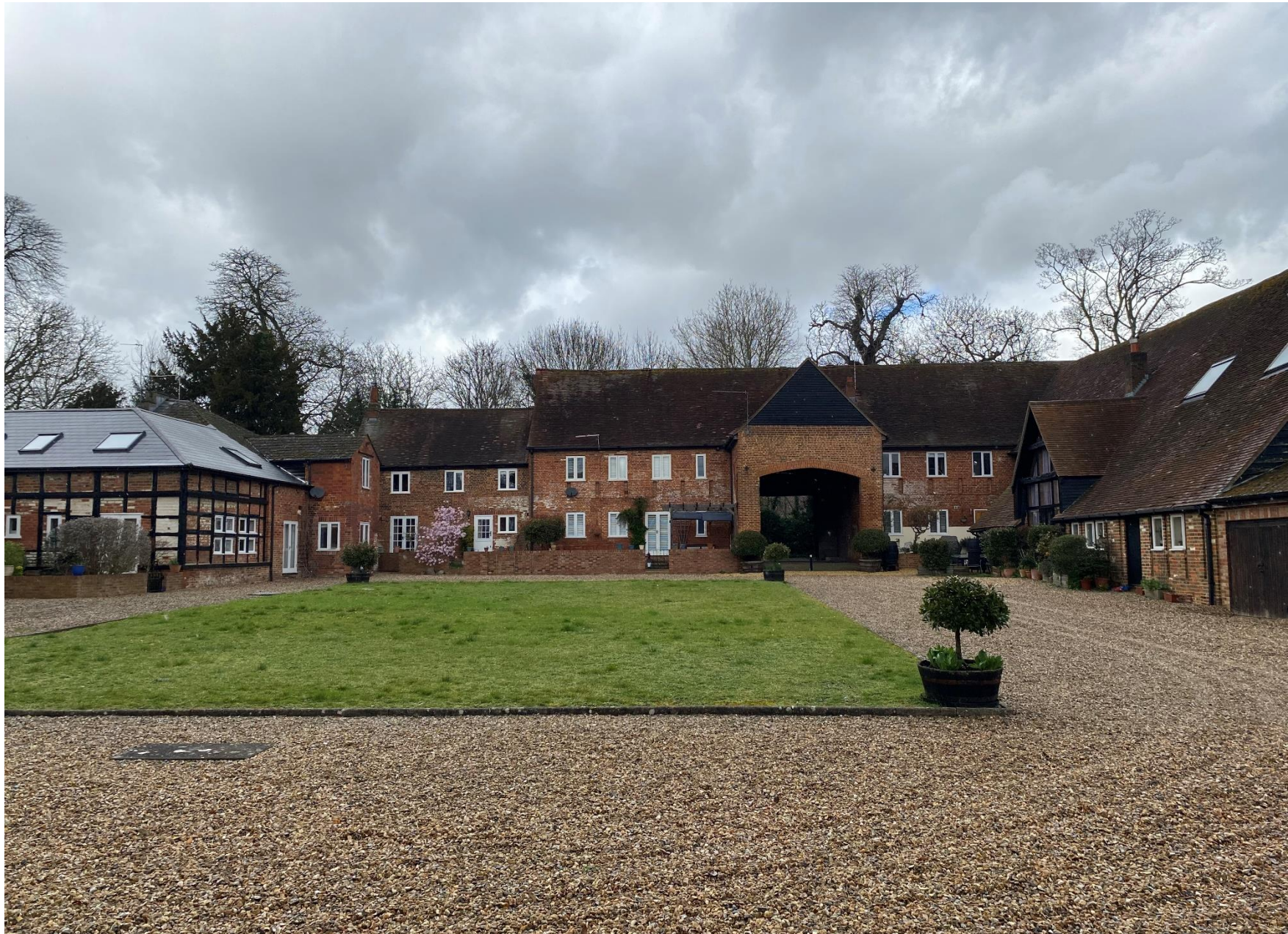
Figure 18 – Closer view of the historic farmstead. The main farm dwellings and barns have been converted into residential. This was carried out in 1986 and involved the conversion of the Site.
