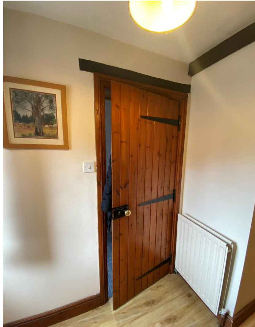
Figure 7 - Main entrance to the relevant area of the Site. Note the timber beam framing extending to the area and use as door lintel.
