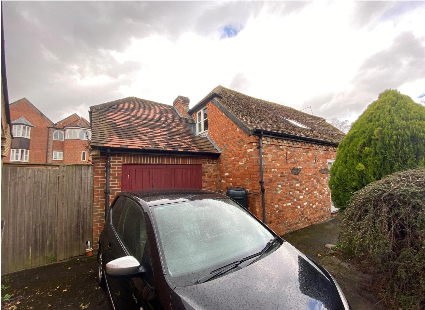
Figure 14 – The Site's east elevation. The later garage extension (which is now in use as the kitchen) is clearly visible.
