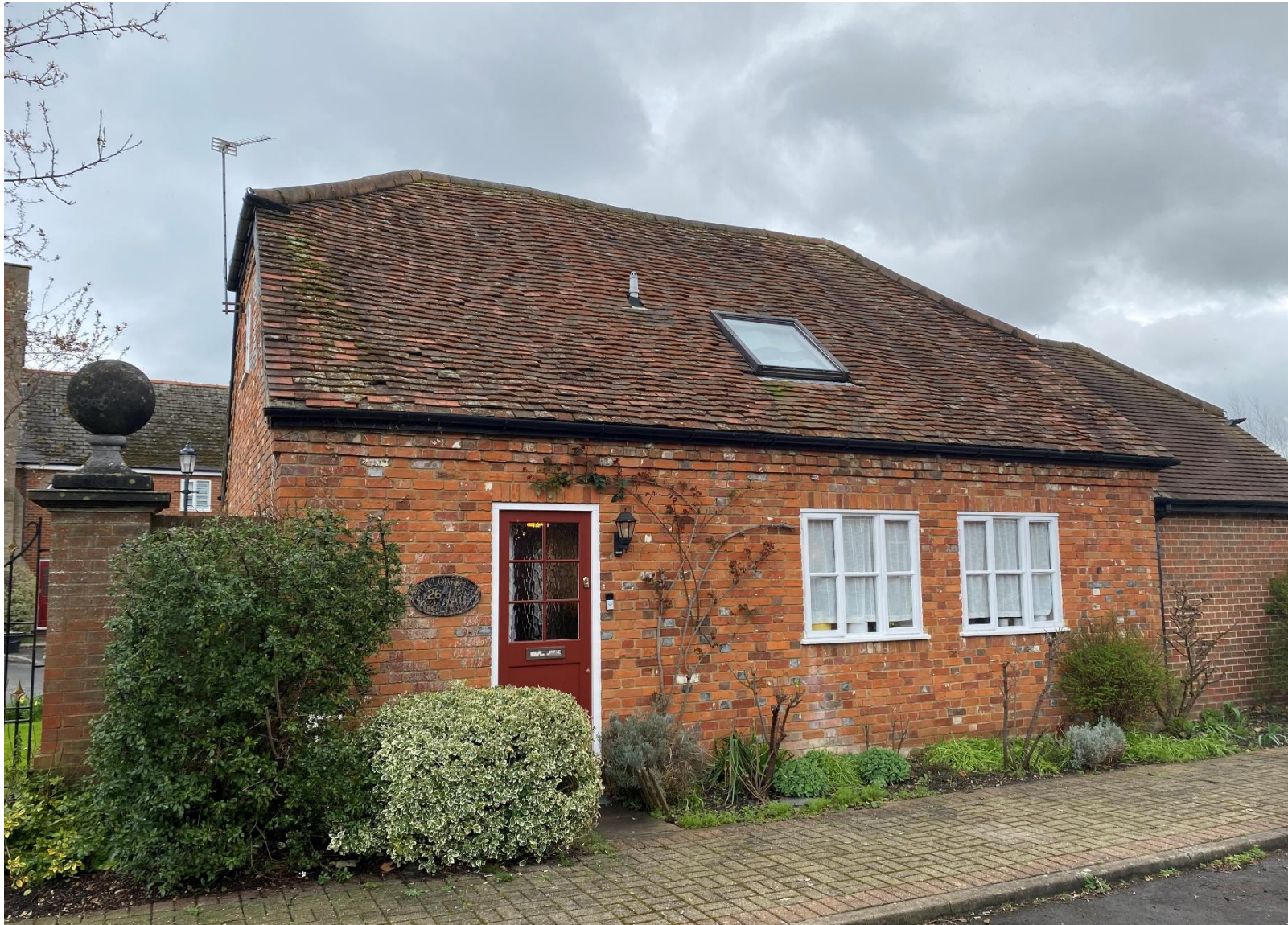
Figure 12 – Western elevation of the Site. The later garage (now in use as kitchen) is viewable on the right.
