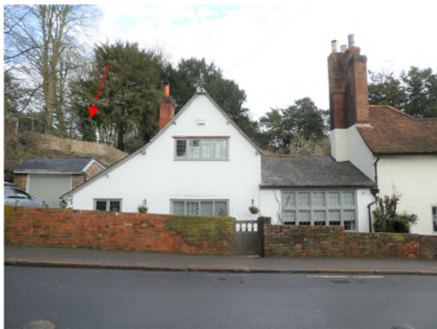
Figure 2: Existing wattle fence to the rear of the garage
