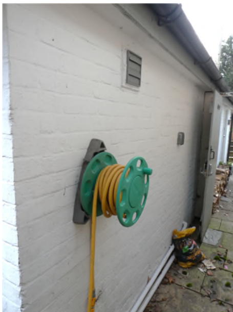
Figure 5: Corner section of wall that has approval for removal and the area leading up to the garden gate that is proposed for removal
