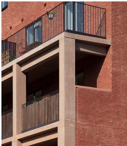
Henley Halebrown Chatt Court PreCast Deck
