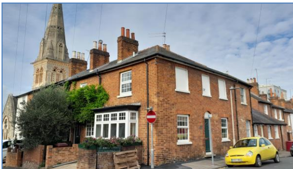
Fig 1. 2 Beehive Cottages as viewed from St Johns Road. Photo taken by case officer on 03/10/2022
