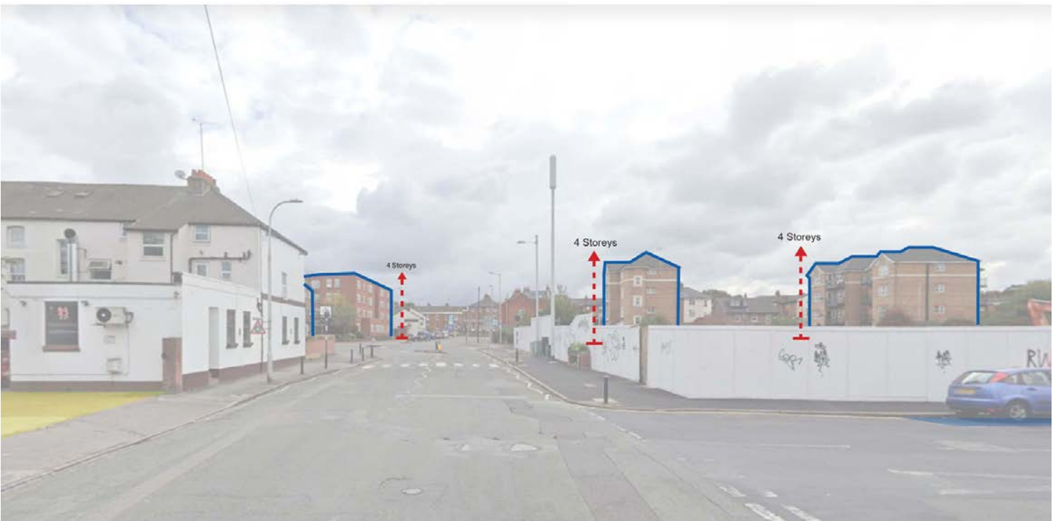
Fig 13: Bedford Road facing south
