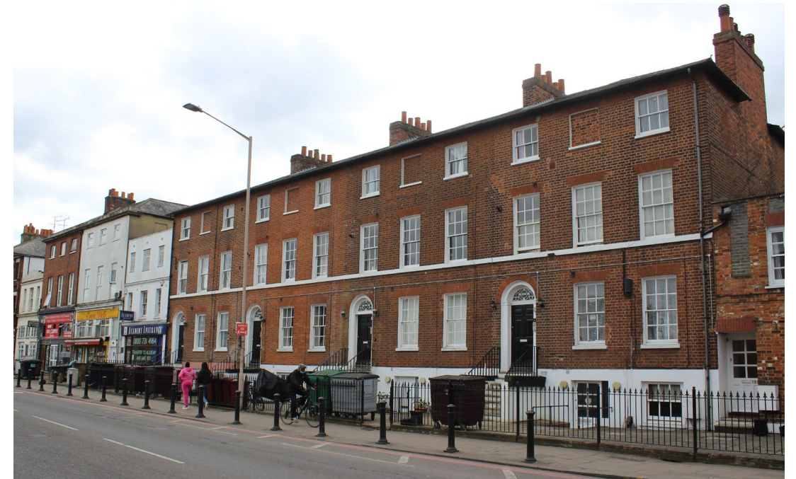
An early / mid-19th century Georgian terrace at Nos. 187-193.
