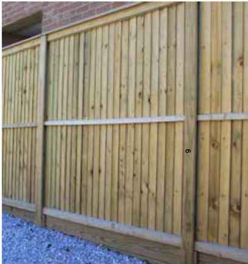
Typical Fence View
