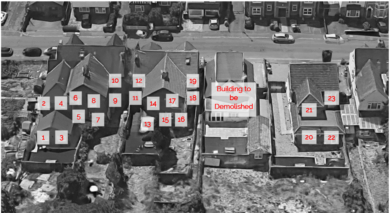
17-27 Newcastle Road (Rear)
