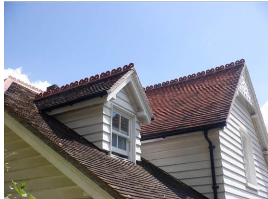
6. Tight timber cladding on dormer and gable.
