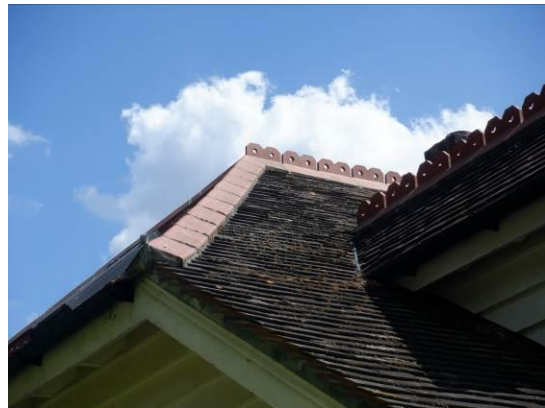
4. Intact ridge and hip tiles and mortar.
