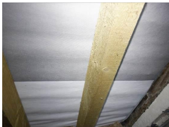
12. Intact non-bituminous (first roof void).
