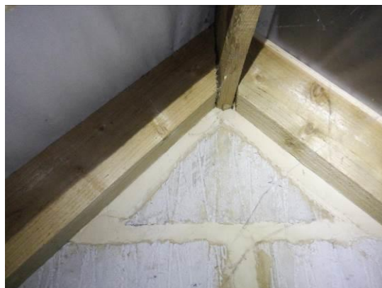
14. Blockwork gable tight to roofline (first roof void).
