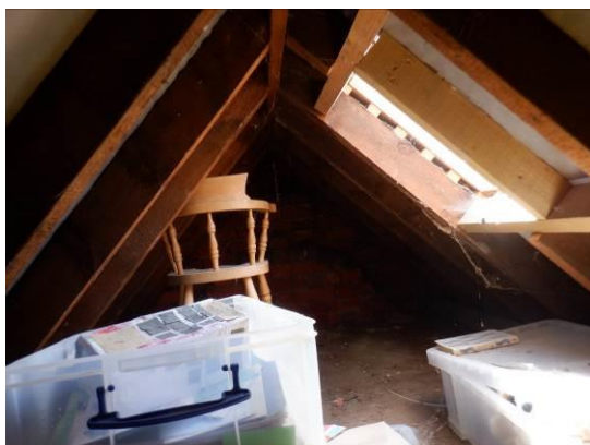
17. Rooflight in void (second roof void).
