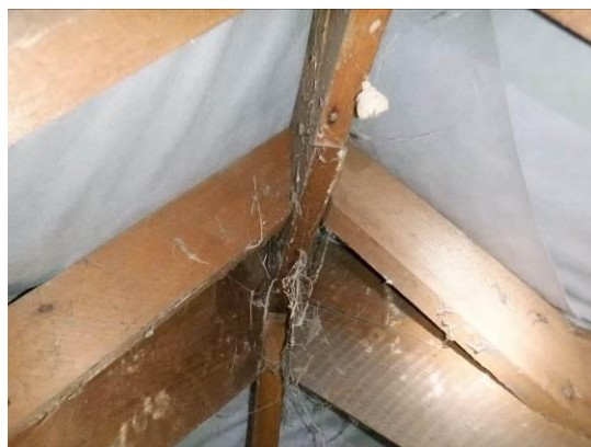
18. Cobwebbed ridge (second roof void).
