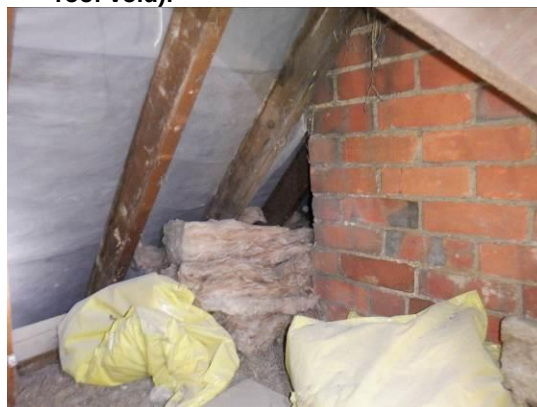
16. Brickwork chimney blocking access to eastern end of void (second roof void).
