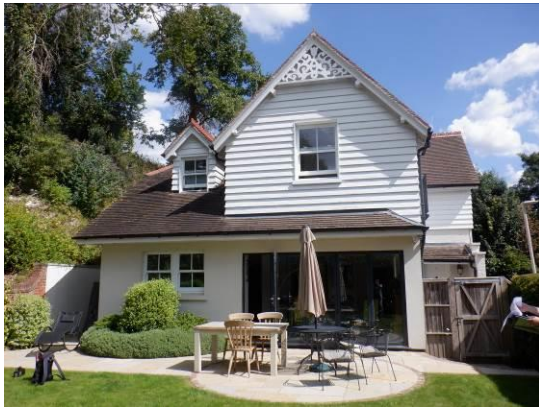
1. Side of the house viewed from the west.
