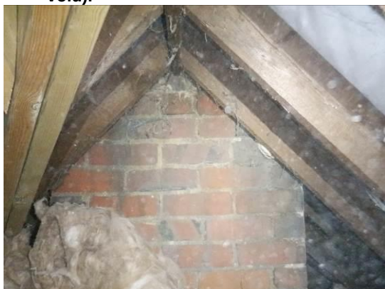
15. Cobwebbed brickwork chimney (first roof void).
