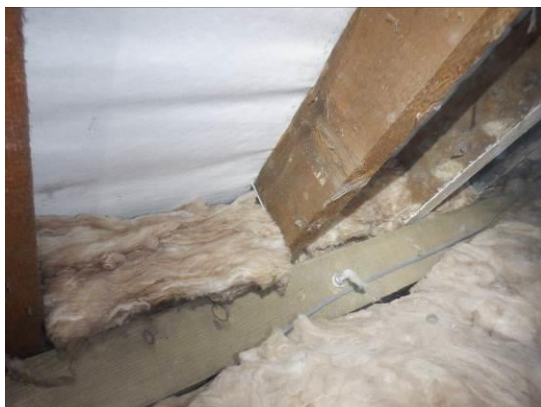
13. Eaves filled with fibreglass (first roof void).
