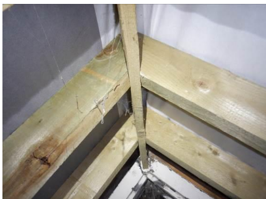
11. Lightly cobwebbed ridge (first roof void).
