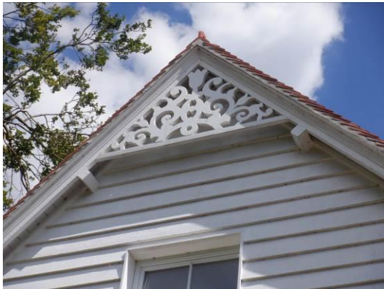
5. Intact verge mortar.
