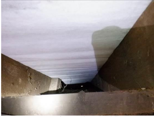
19. Open eaves (second roof void).
