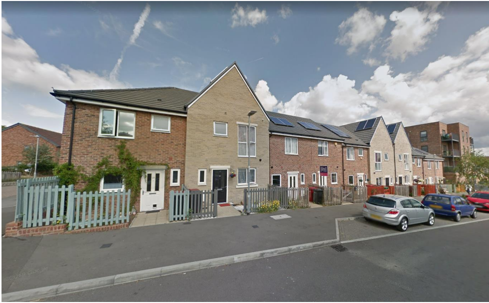
Image 6 - Street view of 23-41 Leven Street
