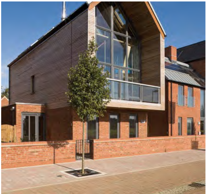
Clay brick paving to house entrances as seen in Upton site C - HTA Design LLP
