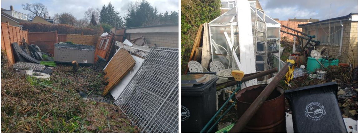
Figures 7 and 8: Debris in northern section next to vegetated areas and greenhouse with surrounding debris, respectively.
