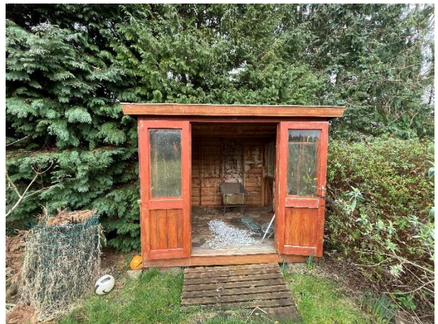
Photograph 12. Outbuilding 2 viewed from the south.
