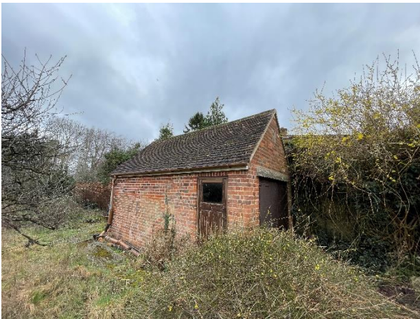
Photograph 9. Outbuilding 1 viewed from the south-west.
