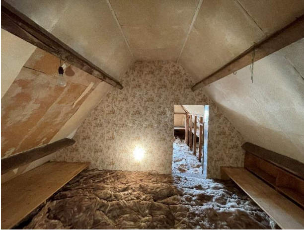
Photograph 7. The central section of the loft space.
