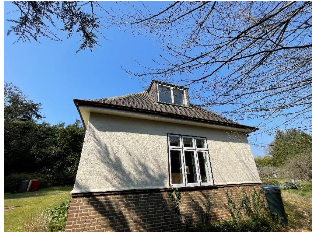
Photograph 2. The eastern elevation of the dwelling.
