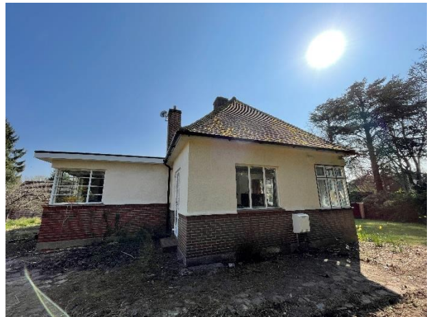
Photograph 4. The western elevation of the dwelling.
