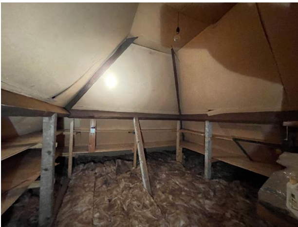
Photograph 5. The western section of the loft space.
