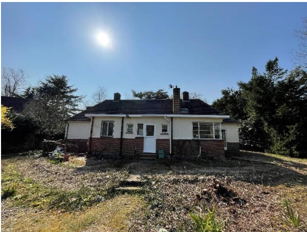
Photograph 3. the northern elevation of the dwelling.
