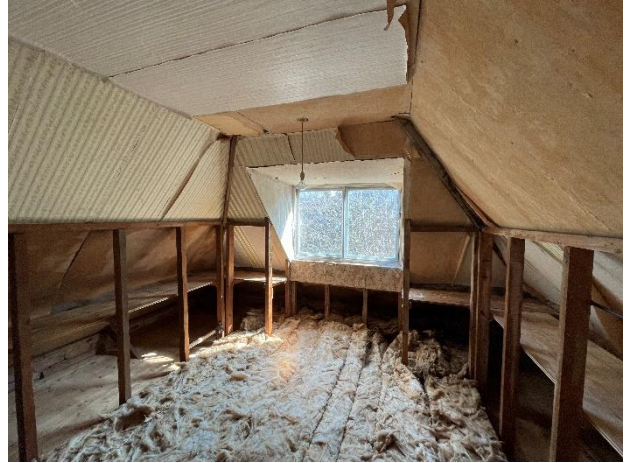
Photograph 8. The eastern section of the loft space.
