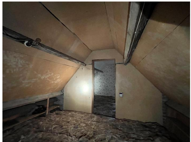
Photograph 6. The central section of the loft space.
