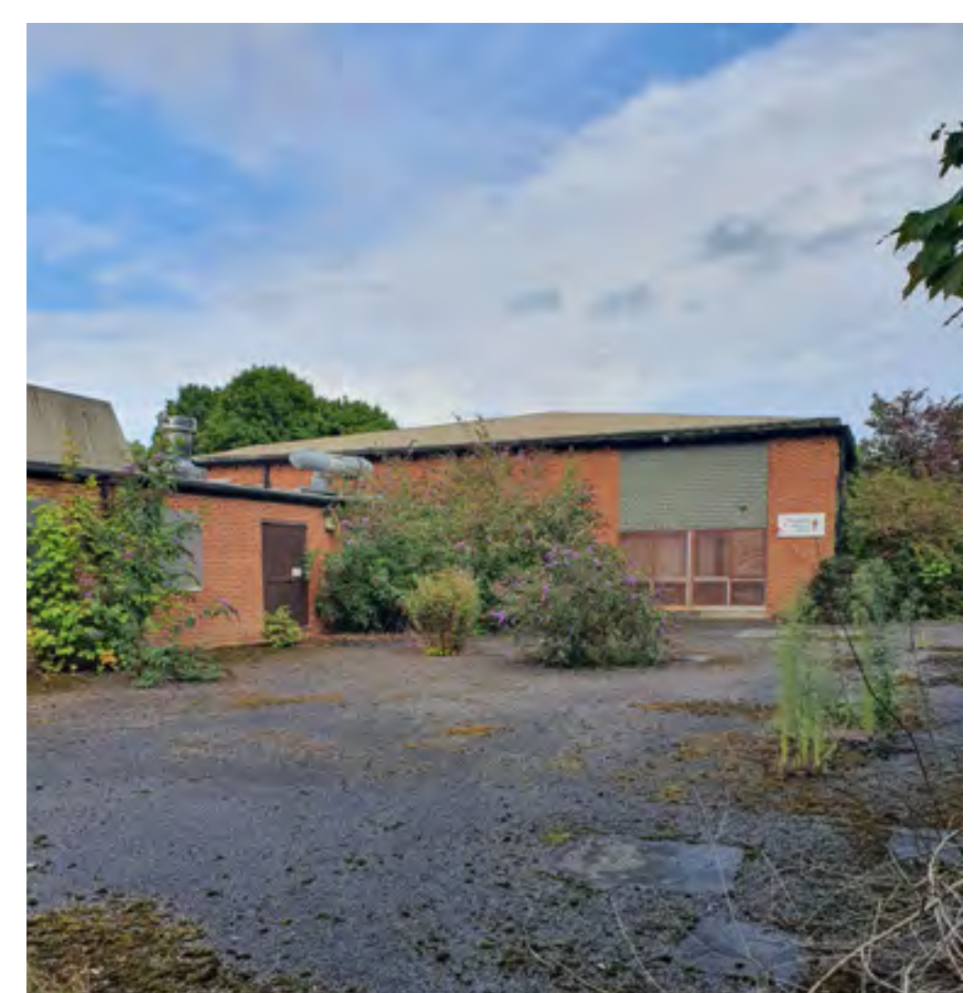
Existing vacant buildings on the site
