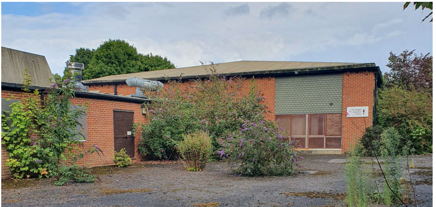
Existing Site Photography - Looking north towards the closed Day Care Centre
