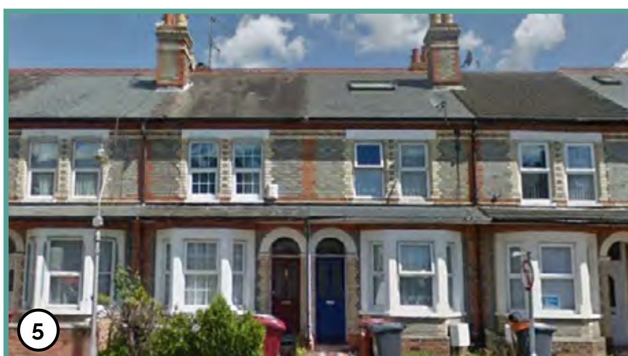
5 Paired first floor windows
