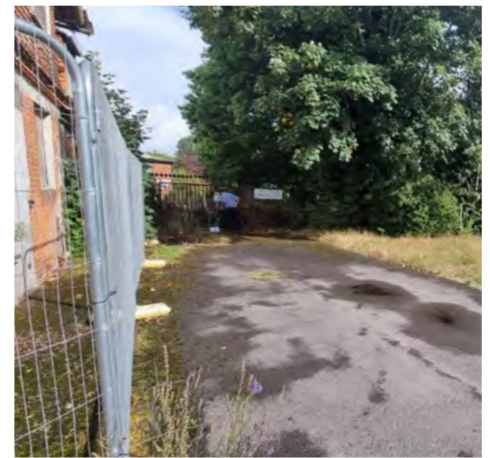
Existing site entrance on Amethyst Lane
