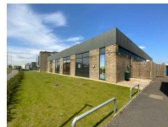
Recently refurbished commercial unit the other end of Portman Road using glazing and brick with cladding parapet.
