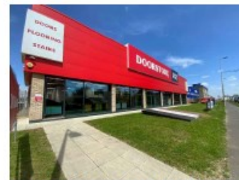
Industrial unit using the synthesis of brick shop front at ground floor and cladding to the first floors. A similar material approach will be used in the proposal for 60 Portman Road.
