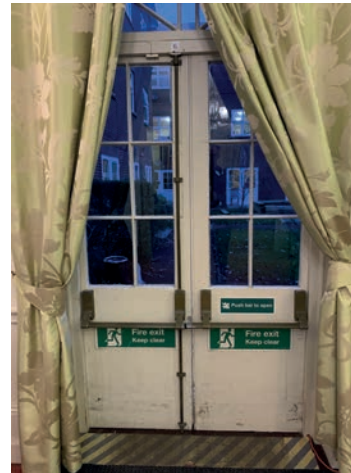
3 Existing Doors - internal view
