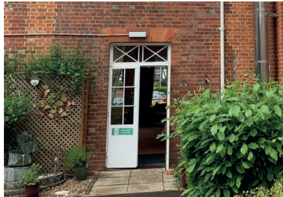
1 Existing Doors - external view
