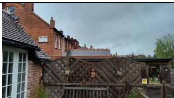
Fig 1. Rear of 4 Kidmore Road looking out towards 6 Kidmore Road
