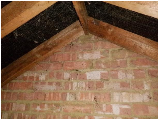
17. Brickwork gable with intact mortar (roof void).
