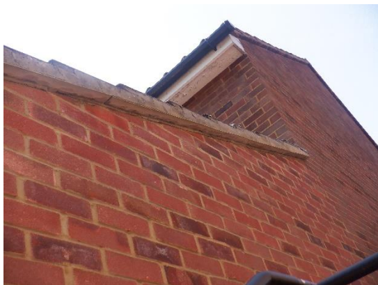
5. Intact verge mortar (north-western elevation).
