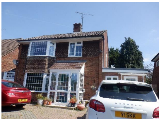
1. Front of the property viewed from south-west.
