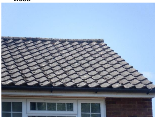
3. Tight interlocking roof tiles (rear elevation).
