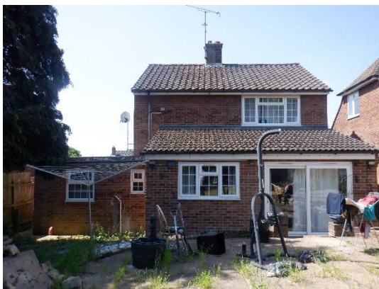
2. Rear of the property viewed from north-east.
