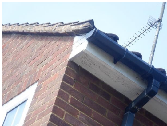
7. Timber soffit tight to brickwork (rear elevation).
