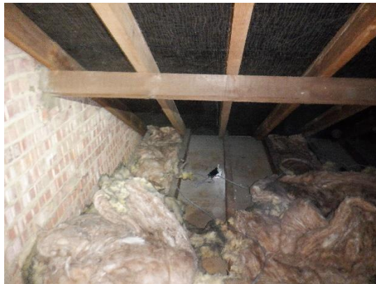
16. Fibreglass insulation throughout, open eaves (roof void).
