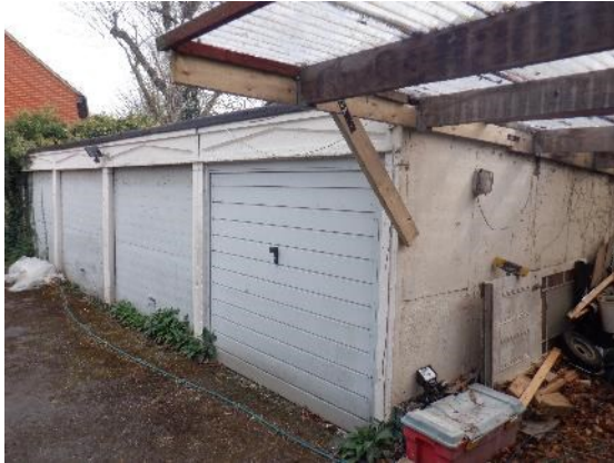
1. Front of garages viewed from north.
