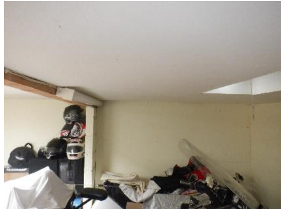
10. Stored items in front of plastered over garage doors.
