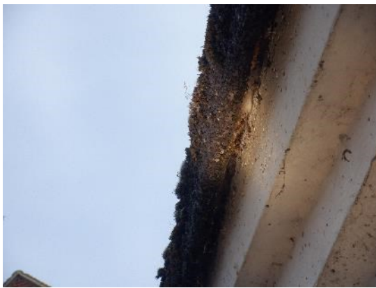
3. Bitumen roofing felt covering roof (front elevation).
