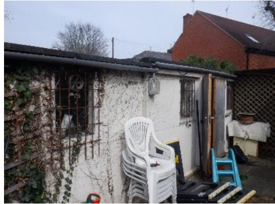
2. Rear of garages viewed from south.
