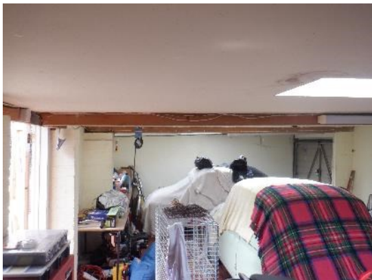
11. The ceiling and walls were fully plastered internally.
