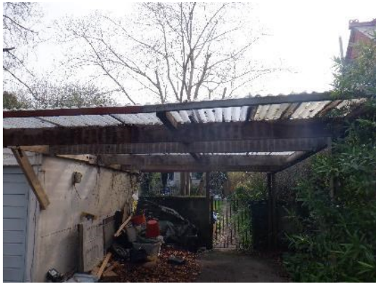
7. Corrugated plastic sheeting above timber framed lean-to at the western end of the site.
