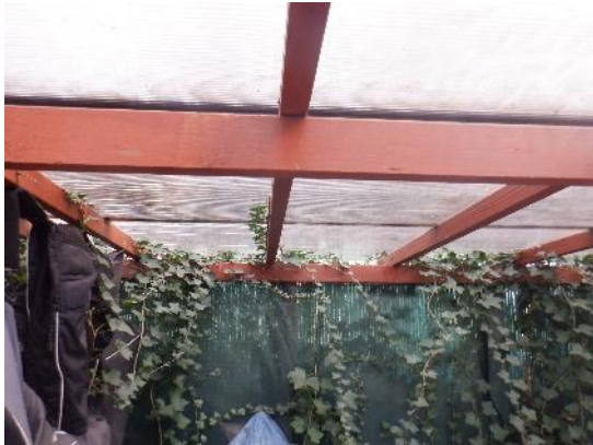
9. Corrugated sheeting above timber framed storage shed.
