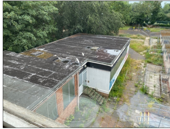
Photograph 18. Eastern rear extension
