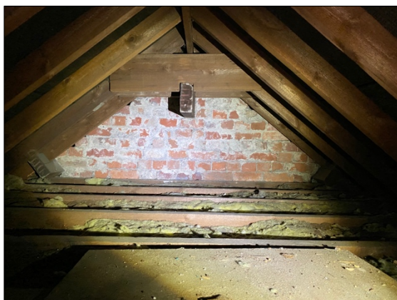
Photograph 19. Example of one of seven roof voids
