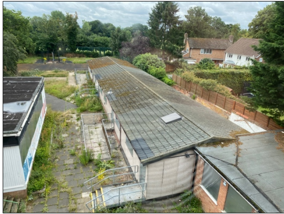
Photograph 17. Western rear extension
