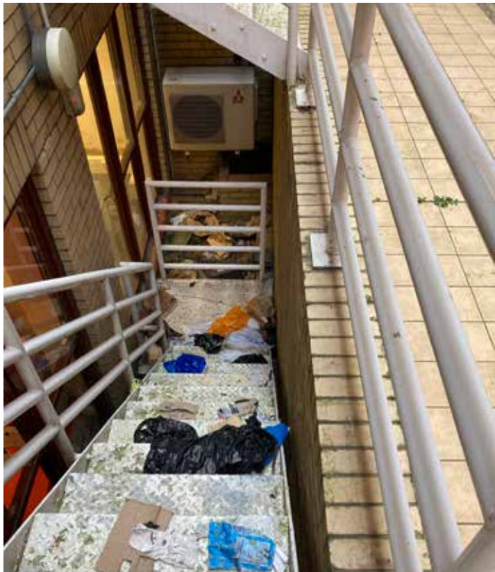
Fire escape stairs from rear of basement
