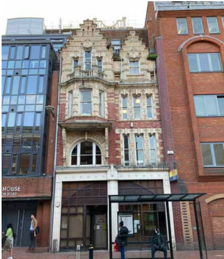
Two main entrances at front elevation
