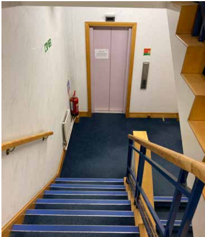
Access route to the other floors
