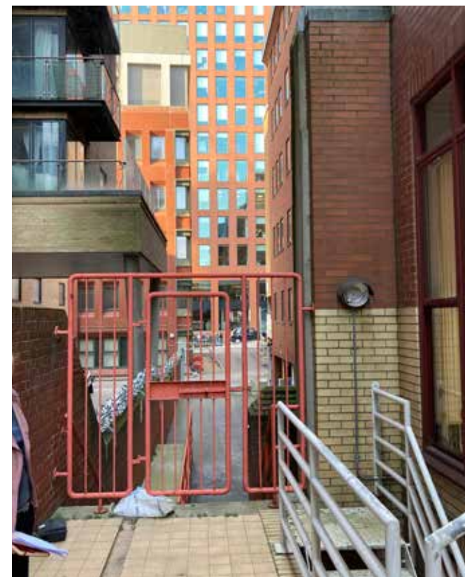
Secure access to the back of the building
