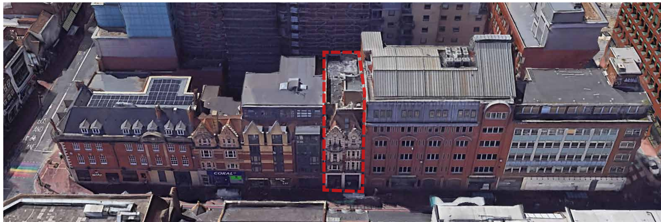
Overhead view of the site looking west
