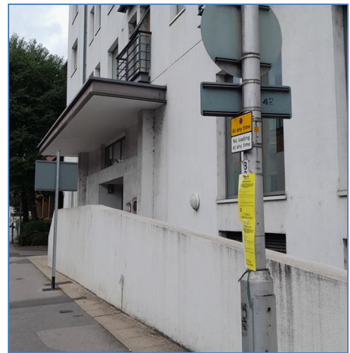
Fig 2 - Photograph of the existing front of 47 Queens Road taken by case officer on 30/09/2022
