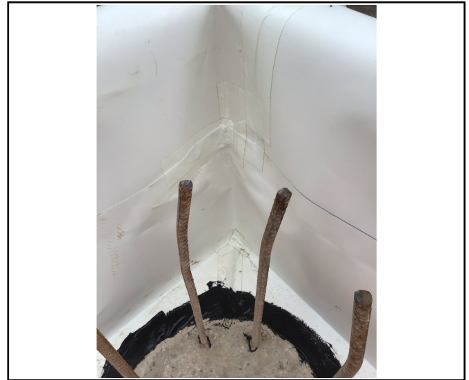
Reinforced corner detail.
