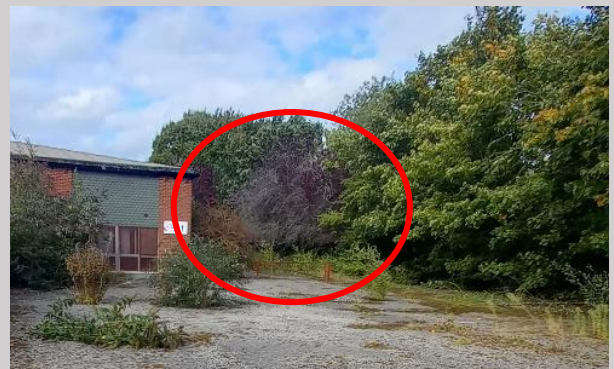
Photograph 4: H2 from the south
