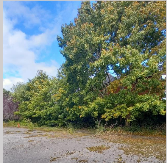
Photograph 2: LT2 from south west
