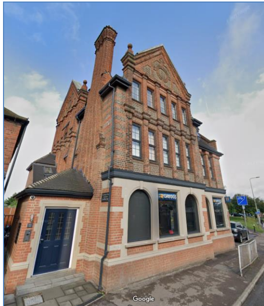
Fig 1. Front of 72 Whitley Street. Image captured in August 2021. Image retrieved from Google Street View on 13/04/2023.
