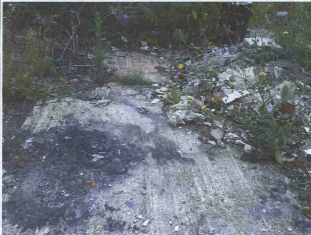
Area used for burning waste towards the east of the site.
