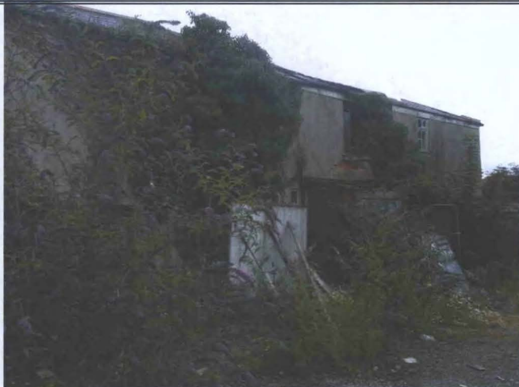
Disused terraced houses trending north-south along the eastern site boundary.
