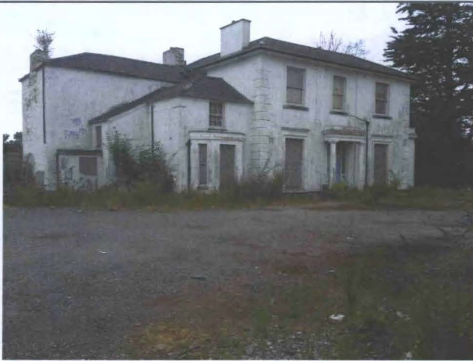
Three-storey Victorian house towards the centre of the site.
