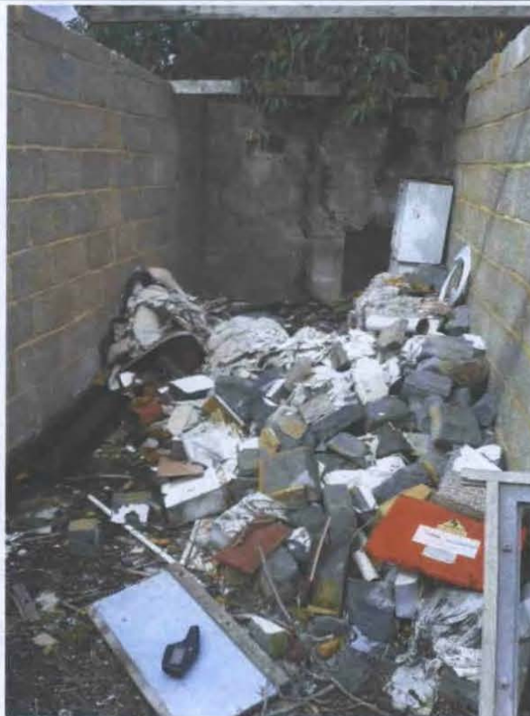
Disused garages typically used to store building materials.
