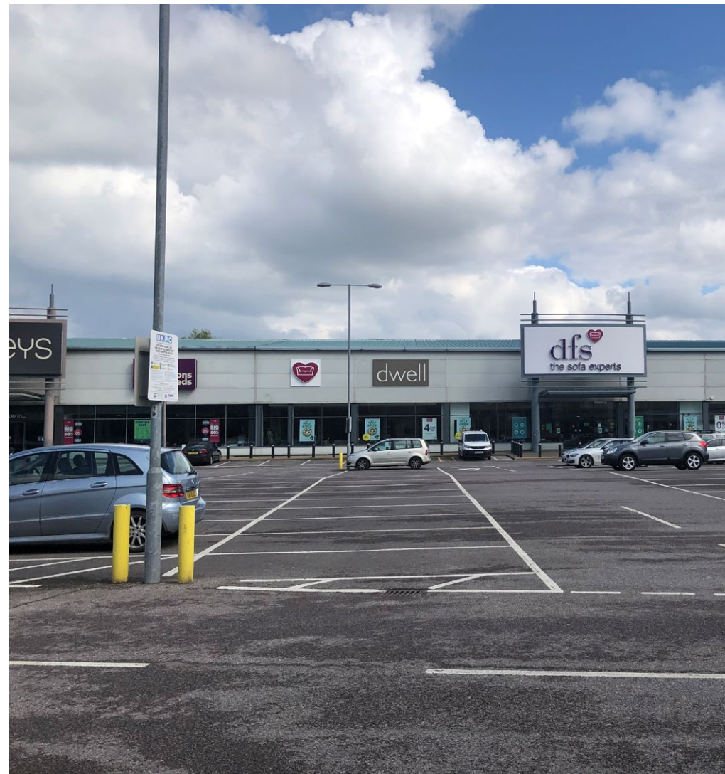
2. Forbury Retail Park - view towards existing building
