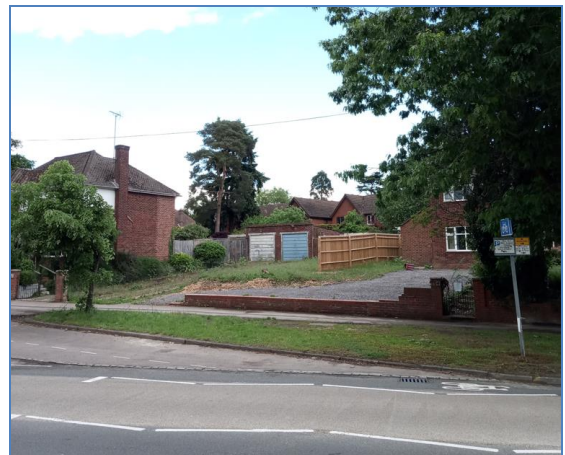
Fig 2. Existing front elevation. Site photo taken on 20/05/2022.
