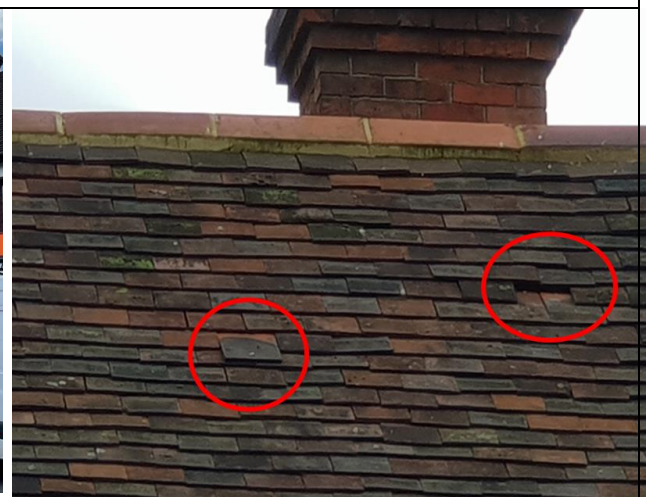
Fig. 4: Some minor repairs to be finalised, for the replacement roof tiles.
