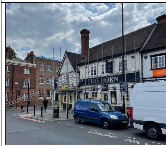
Fig. 3: Scaffolding for Roof Works
