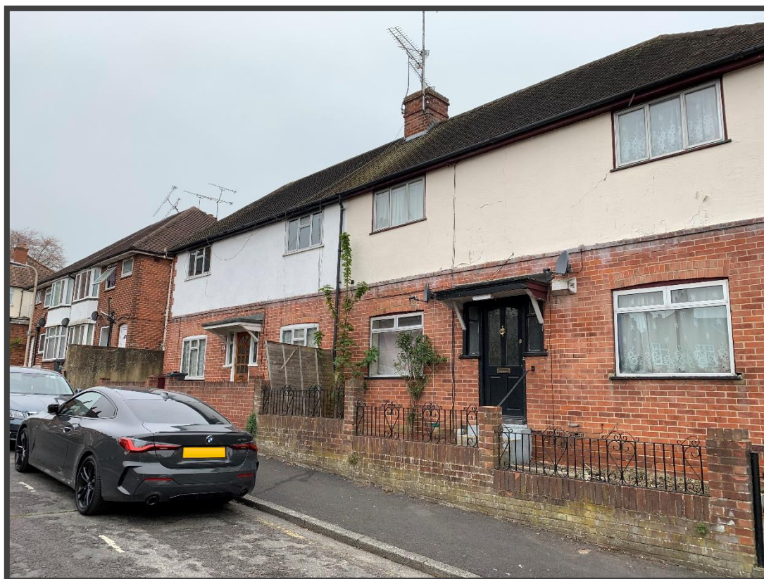
2. 66 - 60 Goldsmid Road - frontage
