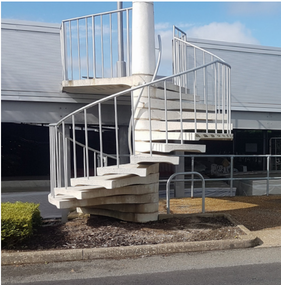
Figure 1-6. View 3 - Car Park Spiral Staircase
