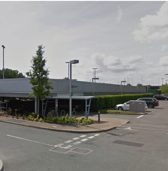
Figure 1-4. View 1 - Approach to Decked Car Park
