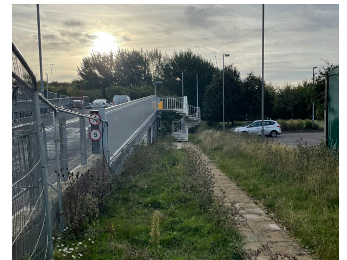
Figure 1-17. View 9 - Rear pathway and spiral staircase adjacent to decked car park
