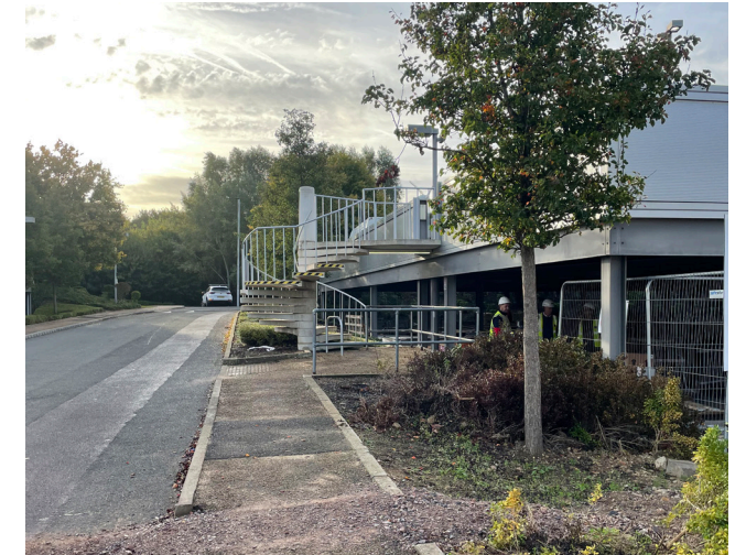
Figure 1-15. View 3 - Existing spiral staircase and pathway adjacent to decked car park
