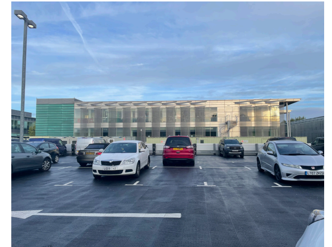
Figure 1-16. View 6 - First floor of decked car park
