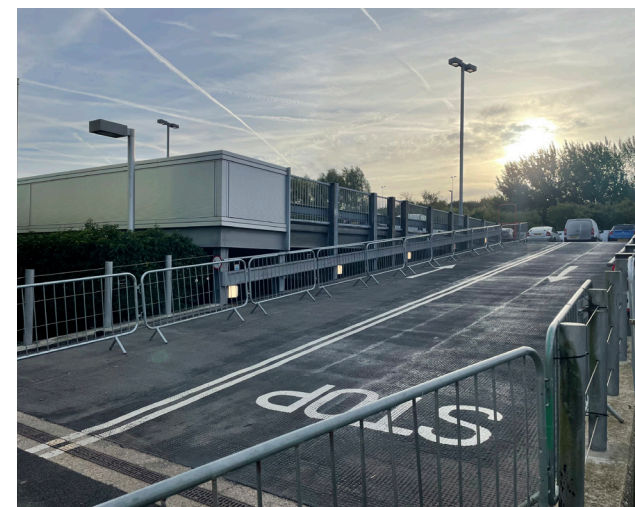
Figure 1-14. View 8 - Ramp up to first floor of decked car park
