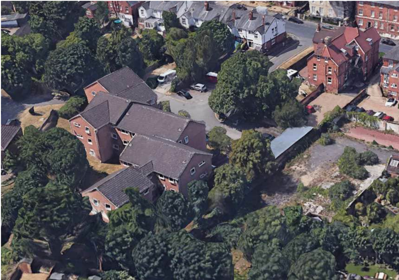
4. Aerial view from the South East
