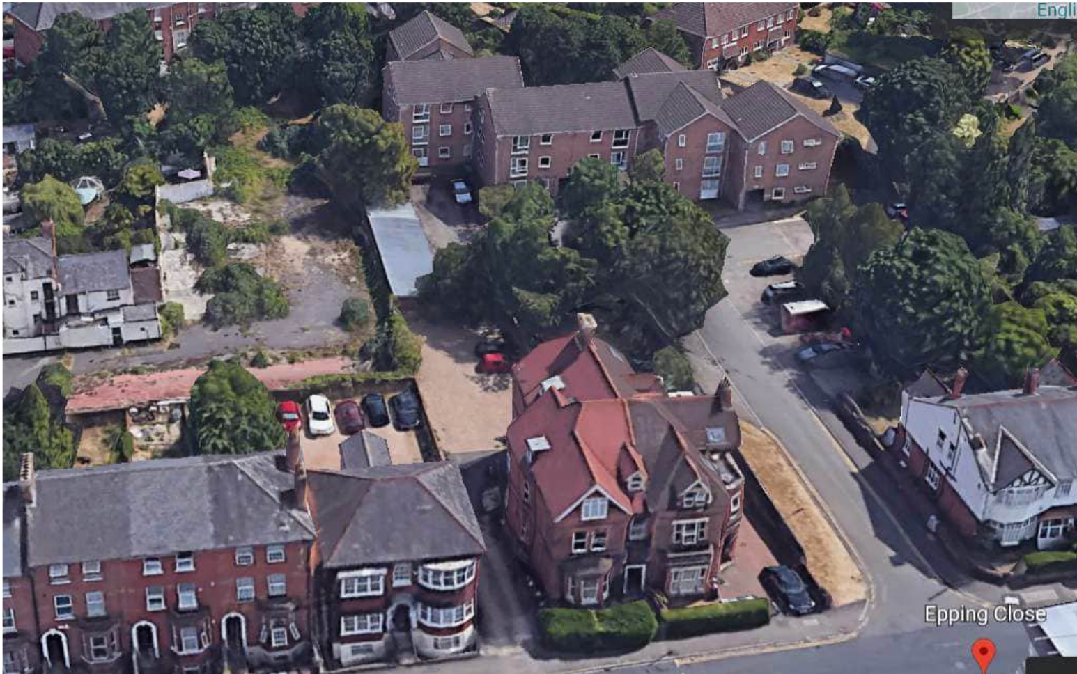
3. Aerial view from the West
