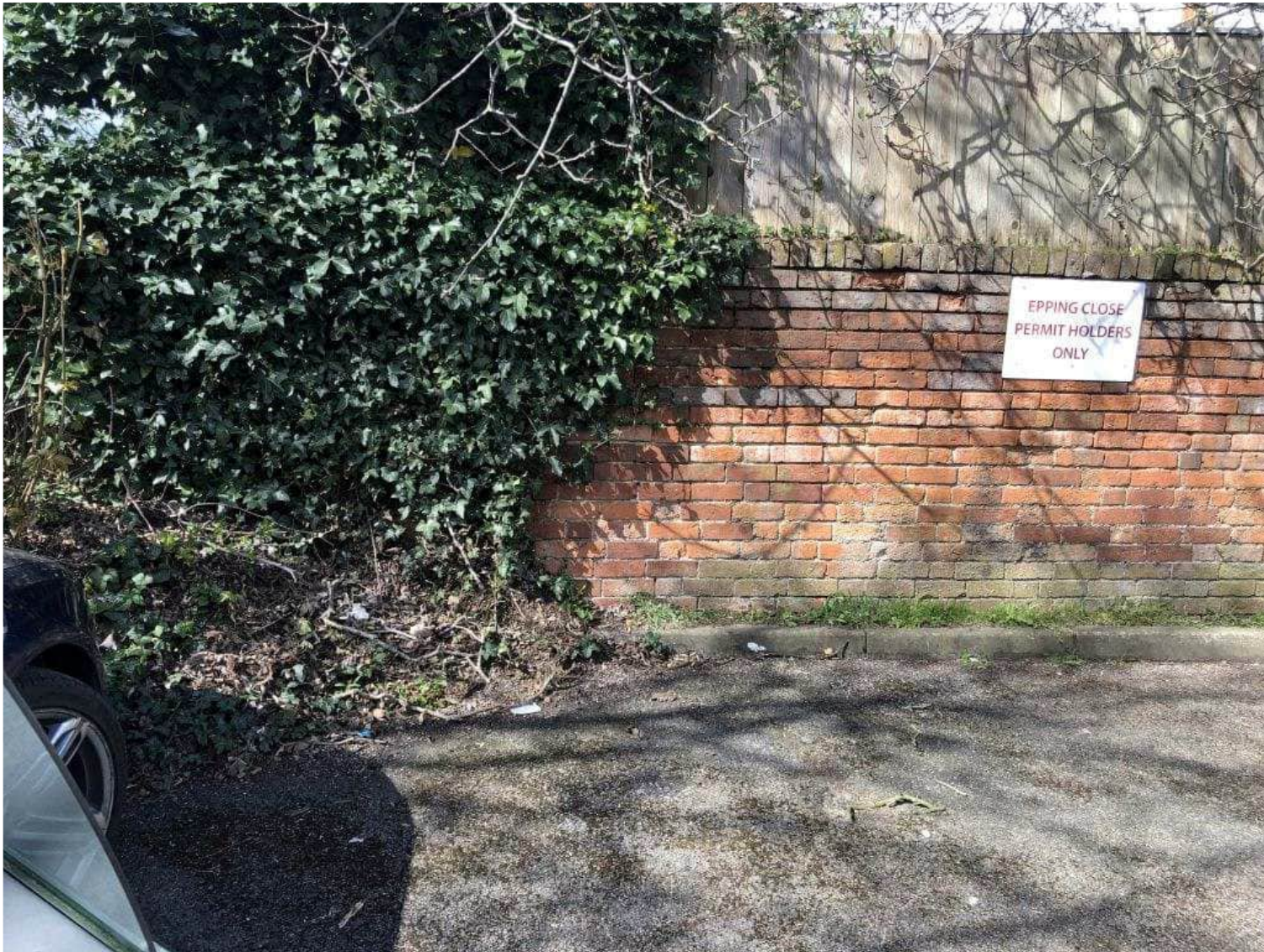
6. Photo showing the boundary wall on East side.
