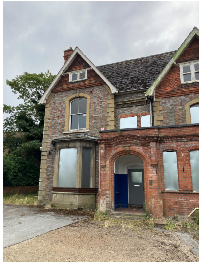
Existing Site Photos
