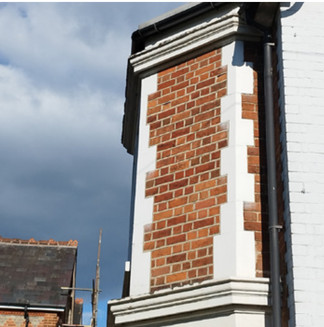
Brick detailing to 10 Brunswick Hill
