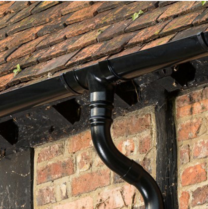
Guttering. Iron fittings
