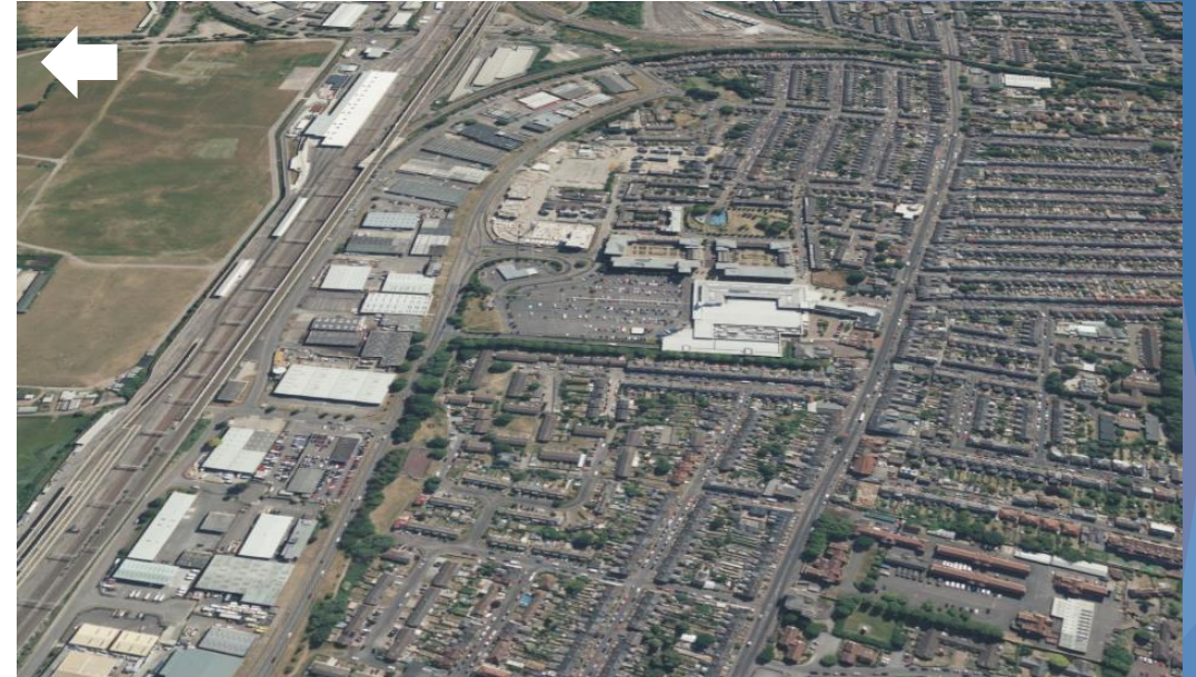
Aerial view of the site looking east
