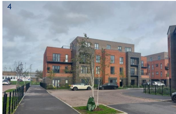
View into the development at the former battle hospital site
