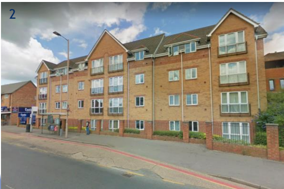
View looking onto existing residential area south of Oxford Road
