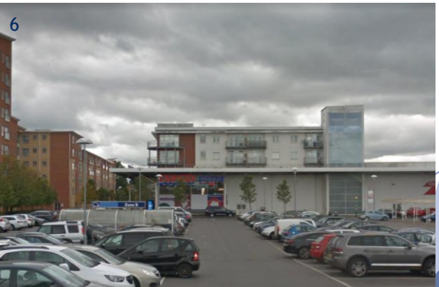
View looking south onto Tesco store
