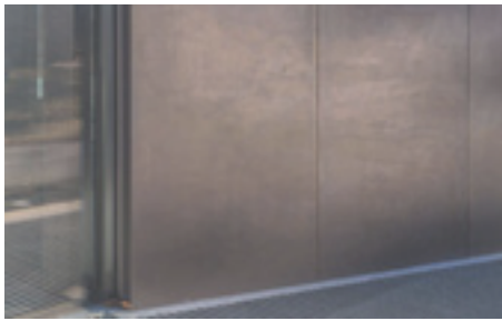
Bronze style metal cladding to in-fill wall sections between new and existing buildings
