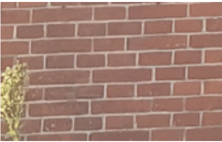
Existing brickwork to the retained existing building
